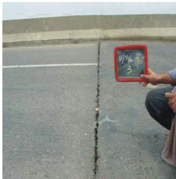
Fig. 2. Joint assembly is removed bridge without joint will not serve properly
