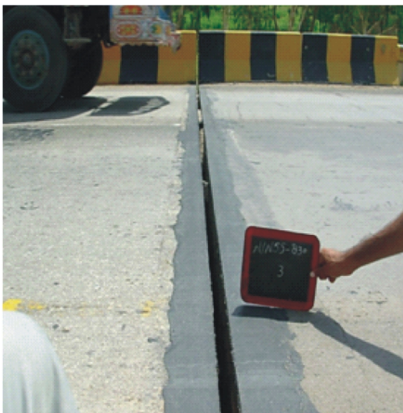
Fig. 7. Neoprene seal removed, gap is being filled with debris
