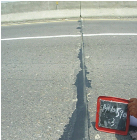
Fig. 6. The damaged wearing course would damage the joint
