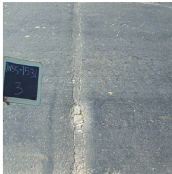
Fig. 9. Improperly repaired joint with bituminous material has restricted the movement
